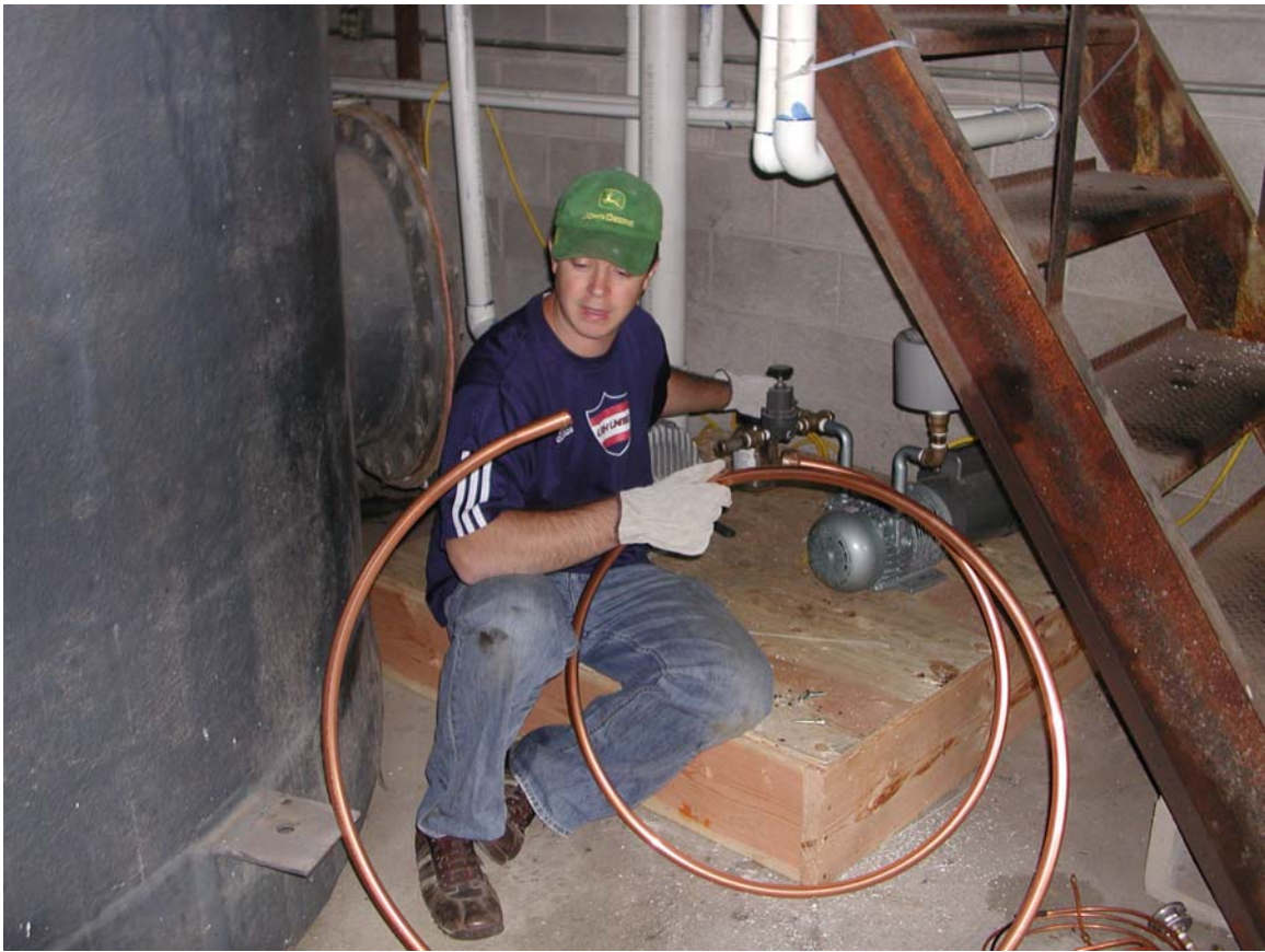
Installing heat exchange piping from compressor
