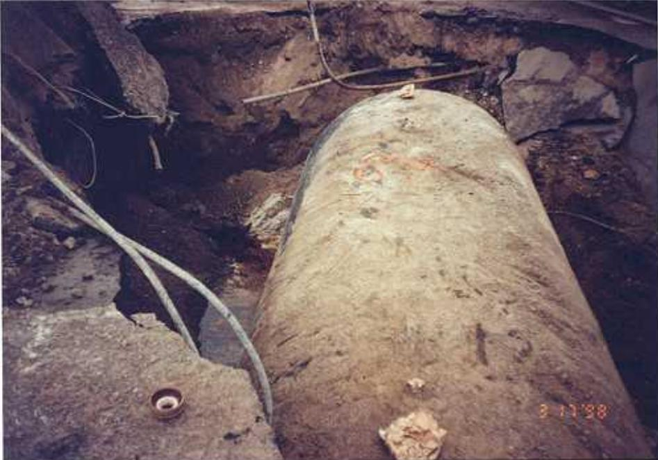
Above: Hydrocarbon sludge floating on groundwater left of the failed underground storage tank.
