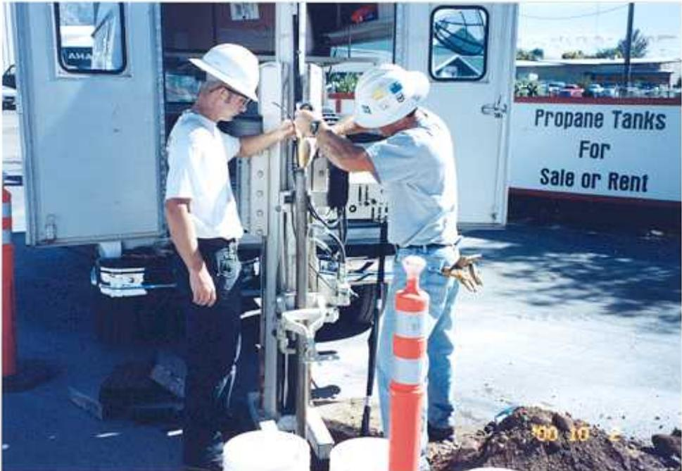
Above: Using a push probe to install the biosparge screens used to inject air (oxygen) into the subsurface soil and groundwater.
